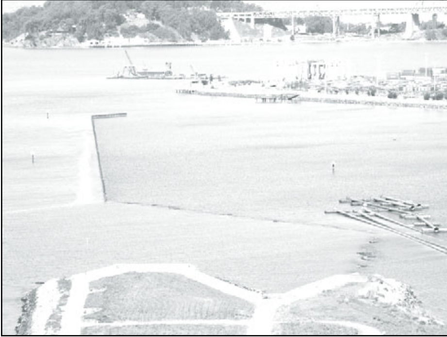
Breakwaters such as this one in the Port of Oakland help protect wetlands created by beneficial use of dredged material ( Photo by Port of Oakland ).
